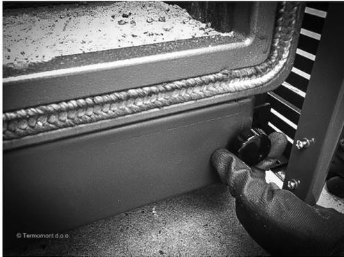
Open the lowest part of the boiler (release the screws).
