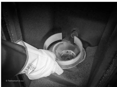
Open the door, release the removable, ring part of the burner.
